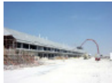
▲ Main Grandstand completed (Top) and in construction (Bottom)
