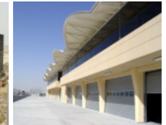
Clockwise from Top: Pit Building; Oasis Complex; ▲ Construction of Media Centre
