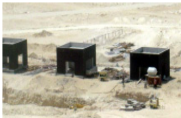
▲ Main Entrance completed (Top) and in construction (Bottom)
