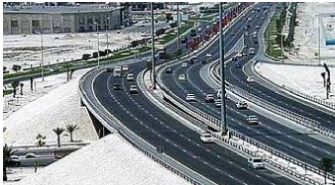
WCT Engineering's RM102mil Al-Seef flyover in Bahrain, completed in 2005
