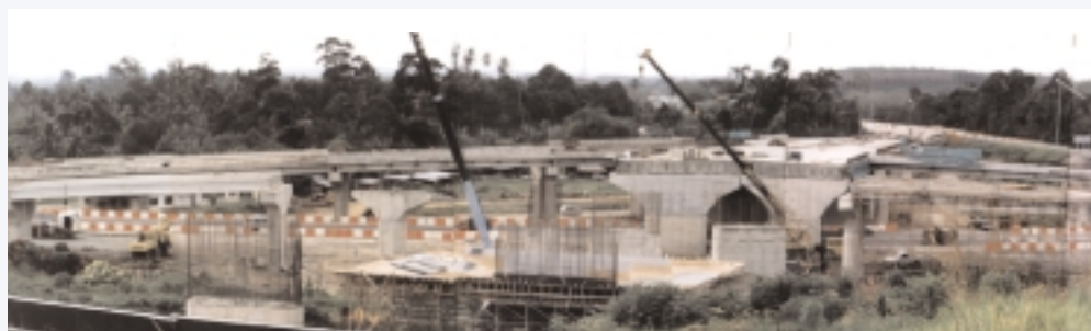
▲ Construction of bridges at Kuala Kangsar Interchange
