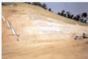
▼ Slope stabilisation works in progress at Lojing - Pos Blau, Blue Valley
