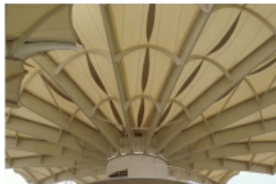
▲ Textile Membrane Roofing of the Canopy Tower
