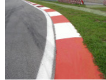
▲ Kerbs - positive, negative and flat kerbs.
