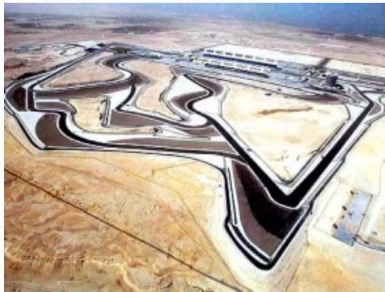
WCT Engineering built the Bahrain F1 circuit together with local partner Cebarco.
