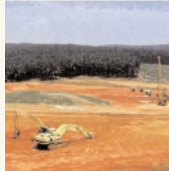
Guthrie Corridor Expressway - Piling works in progress
