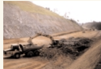
Excavation of rock @ CH 125+300 (east Bound)
