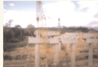
Launching of beams at Bridge over Sg. Bakapor @ CH 114+000
