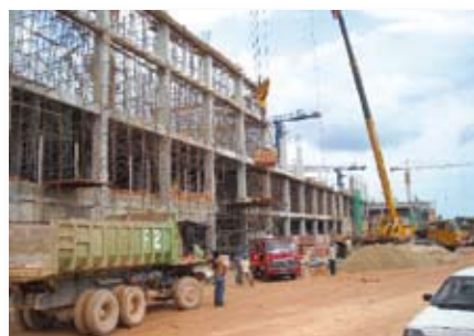
AEON Shopping Mall, Melaka - in progress
