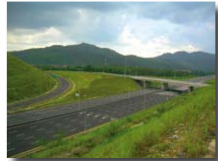
LEKAS Highway – timely completion and delivery of quality works
