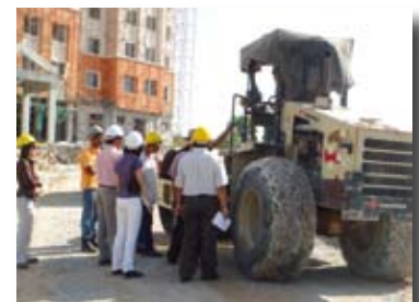
Routine visits to monitor efficiency and quality control at project sites
