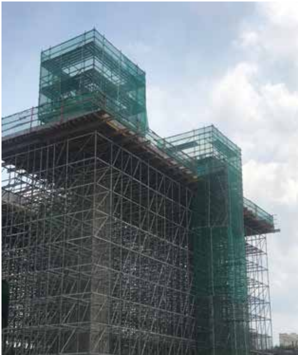
Portal pier cast in situ PERI formwork at MRT V204
