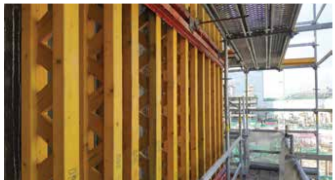
Wall PERI formwork at the mixed commercial development project in TRX
