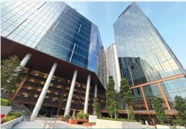
The Exchange TRX Hotel and Office comprises a 29-storey hotel tower and a 13-storey office block.
