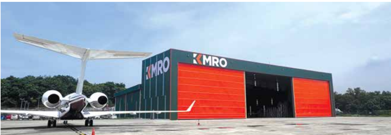
As an integrated aviation facility, SRAC supports tenant operational and expansion needs, including the installation of the first custom-built hangar door for KarbonMRO.
