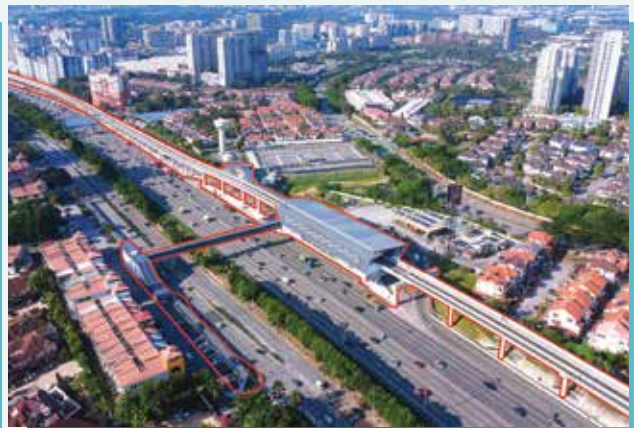
The 5.7 km LRT3 (Package GS02 and GS03) alignment, featuring five long spans and three stations, required meticulous planning and coordination to safely carry out construction across existing rail lines and busy highways while maintaining uninterrupted public operations.
