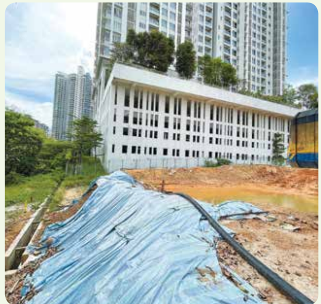
Purpose-built sediment pond at Hilltop 2 project site to filter and treat surface run-off containing silt or effluent before releasing water into the watercourse.
