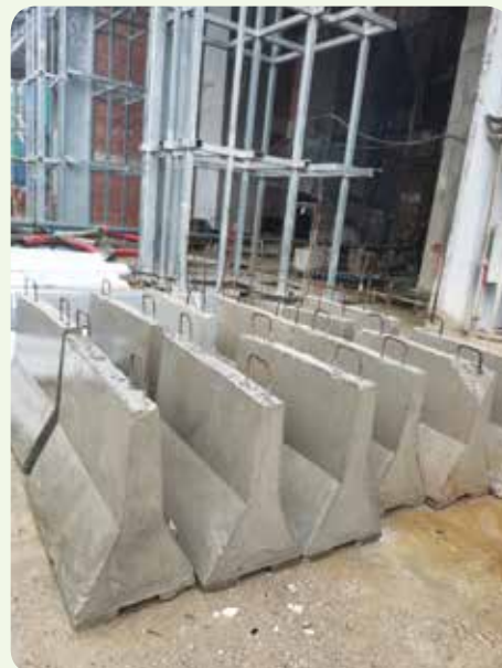
Surplus concrete is used to fabricate road barriers at one of the project sites
