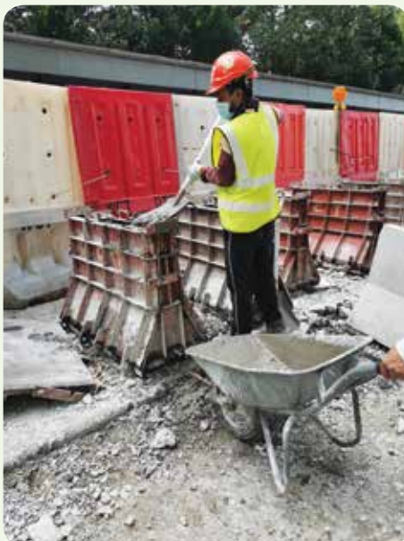
Surplus concrete is used to fabricate road barriers at one of the project sites
